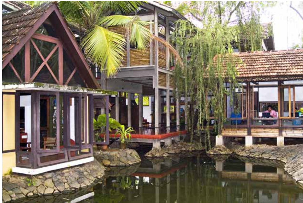
↑ Alternate Methods: The Inspiration Office in Kochi employs a composite system with RCC stilts, combining bamboo and concrete in structures and using ecological materials as much as possible in the moisture and bio-attack prone region of Kerala. (Image: courtesy Inspiration)
