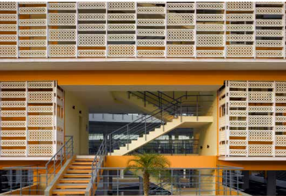
† Intelligent planning: At The Pearl Academy of Fashion in Jaipur, by Morphogenesis, self-shading sliver courtyards keep the sun out and help regulate temperature and daylighting of the study areas. The perforated outer skin is derived from computational shadow analysis, based on the orientation of the façades. (Image: © Edmund Sumner)
