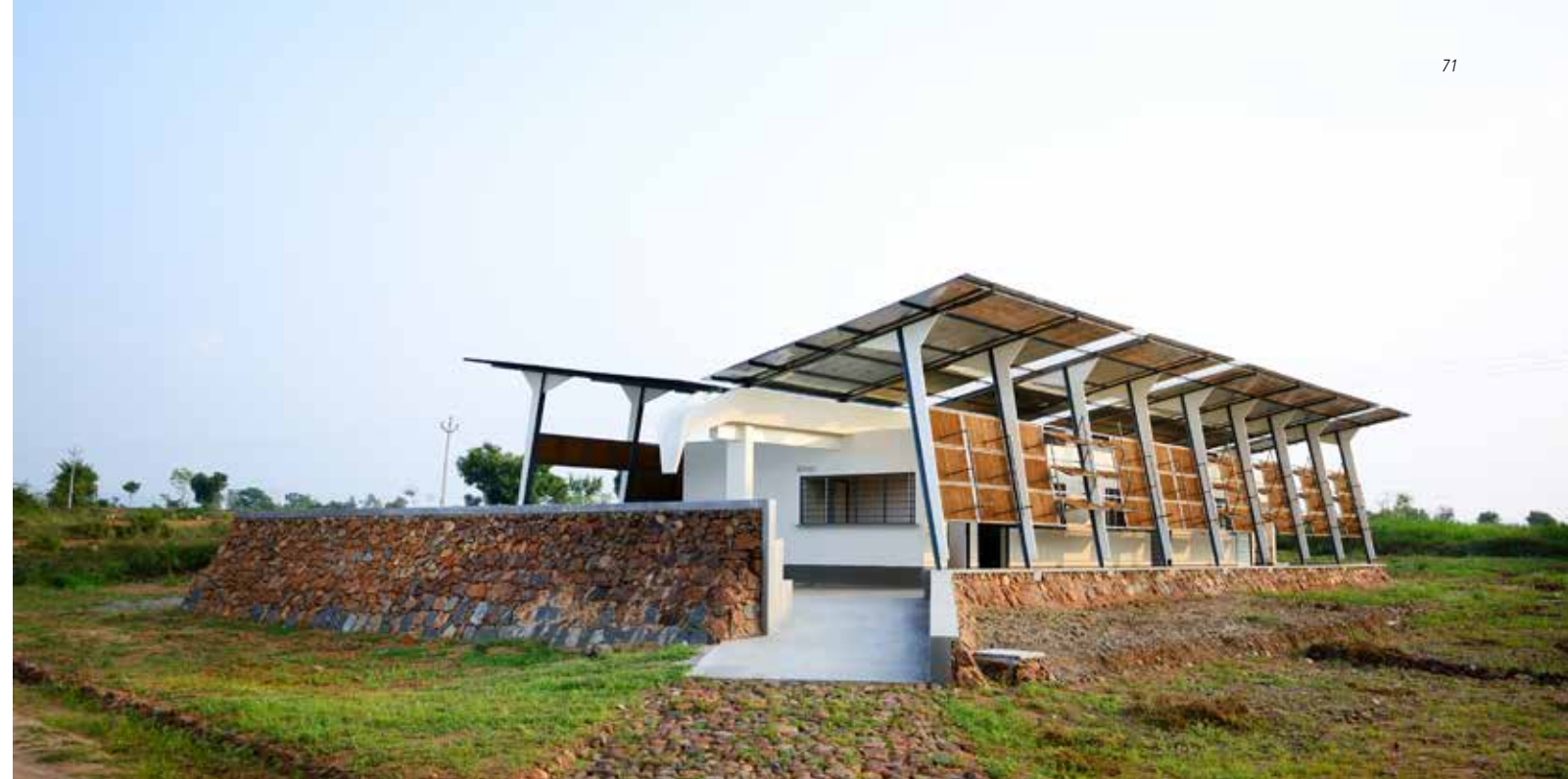
† Intelligent Planning + Innovative Systems: The Primary Healthcare Centre at Dharmapuri by Flying Elephant Studio combines the universal design principle of favourable orientation with the subtle layering of spaces, providing a louvered verandah enveloping the inner building to buffer the heat and sun out. An inverted roof further helps collect rainwater. (Image: courtesy Flying Elephant Studios)
