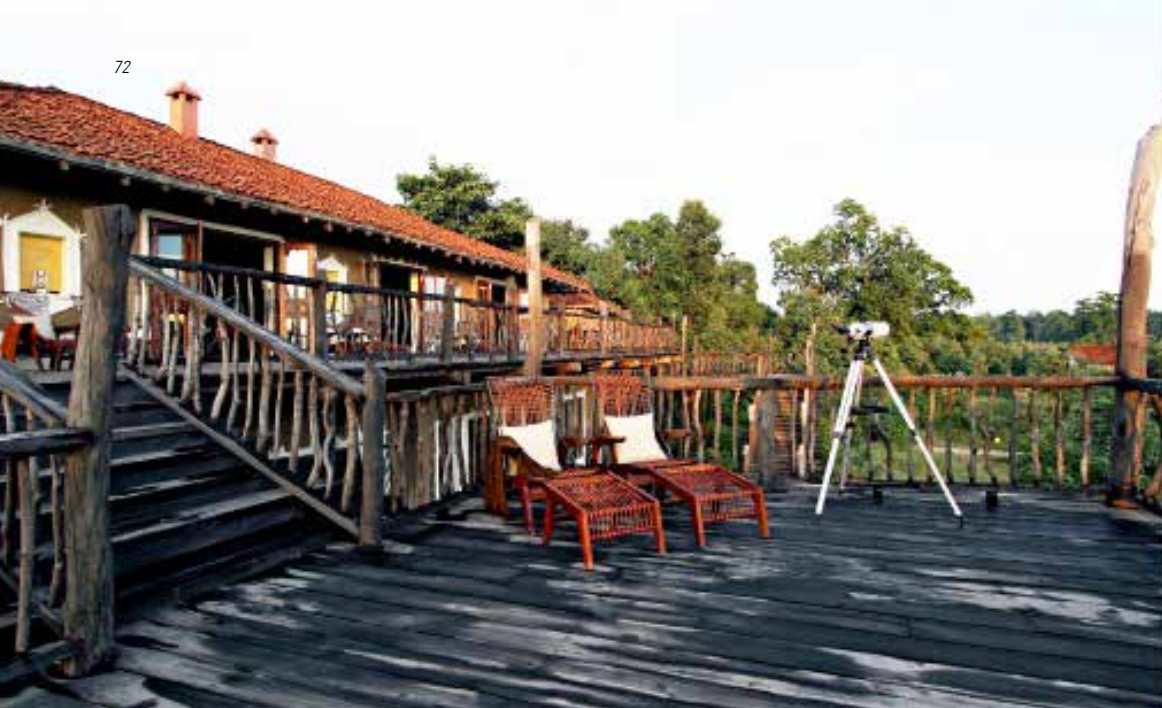
↑ Alternate Methods: The Samode Safari Lodge by Pradeep Sachdeva Design Associates adopts traditional vernacular systems of architecture from surrounding villages and combines this with a Ferrocement skin to reduce the brick and steel used for construction. (Image: courtesy Pradeep Sachdeva Design Associates)
