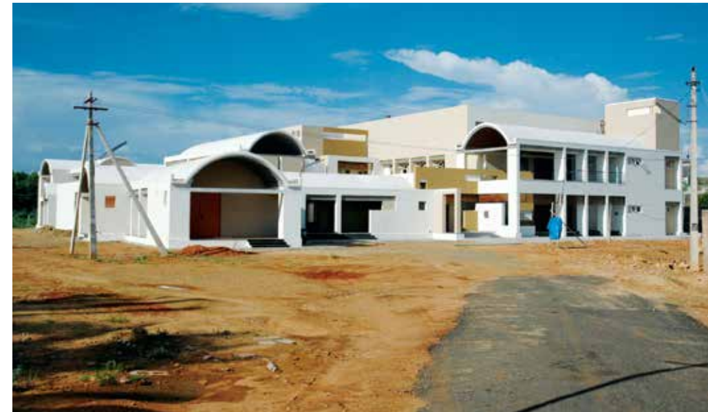
↑ Alternate Methods: The Centre of Hope Orphanage in Chennai is located in the hot and humid equatorial climate of Chennai. It uses shaded terraces, filler slabs and brick vaulted roofing to build within a low budget and yet produce well-ventilated spaces. (Image: courtesy Hundredhands)
