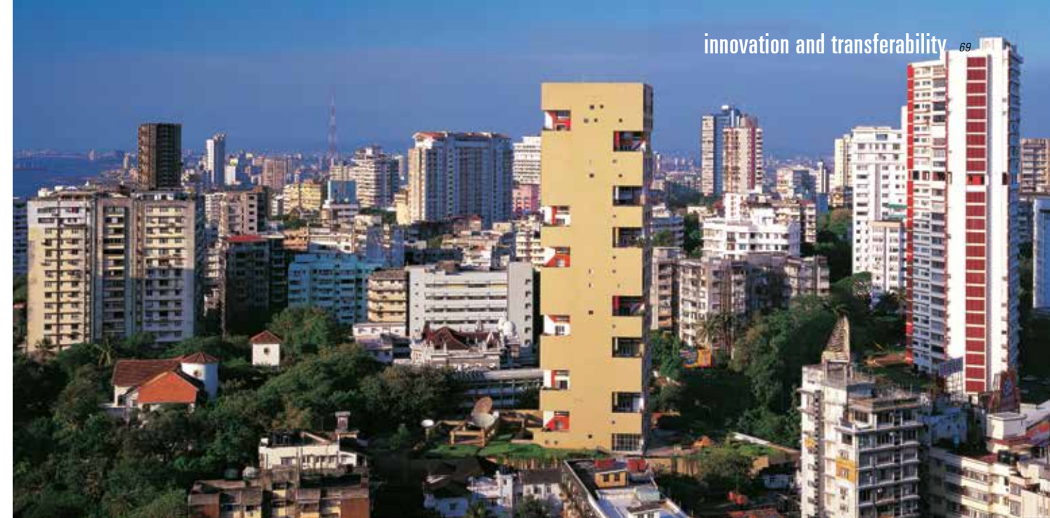
1 Intelligent planning: The Kanchanjunga Apartments in Mumbai by Charles Correa Associates makes use of double-height balconies, a reinterpretation of verandahs, for a layered reading of space that creates comfortable living conditions in the units. (Image: courtesy Charles Correa Associates)
