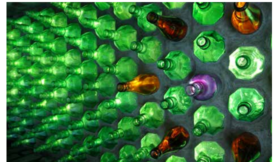
↑ Alternate Methods: The Manav Sadhna Activity Centre embodies experimentation in sustainable architecture, using municipal waste to create filler slabs and walls, scientifically tested to be eco-friendly, providing economical solutions. (Image: courtesy Footprints E A R T H)
