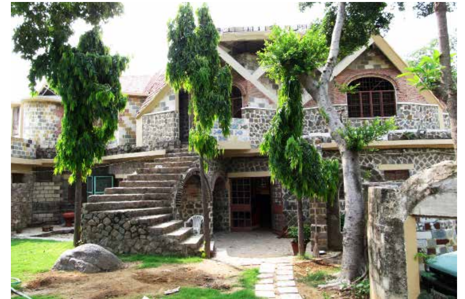
↑ Alternate Methods: The Anangpur Building Centre has time and again been a source of inspiration for site planning and architecture that blends with the ecology of its site. The recycling of materials and alternate construction techniques like vaults, domes and arches rationalise the use and reuse of such architecture. (Image: courtesy Anangpur Building Centre)
