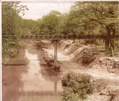
WORRISOME Drainage system of Delhi has raised a lot of stink in recent times.
